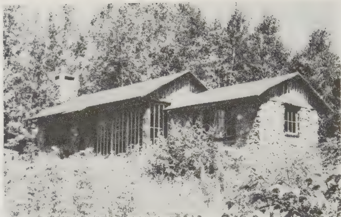
The first completed cabin.
